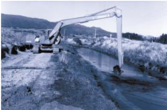
Drain clearing with long-reach excavation.
