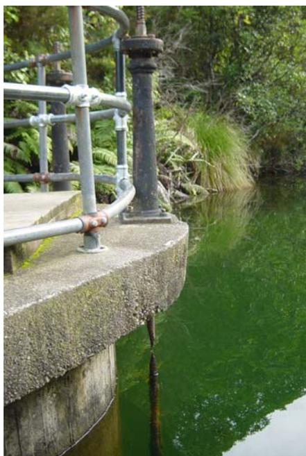
**Fig. C-10:** Intake tower with control valve
