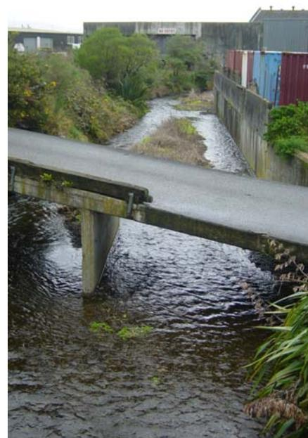
**Fig. B-38:** Korokoro Stream channel parallel to Cornish Street, max design discharge 40 m<sup>3</sup>/s.
