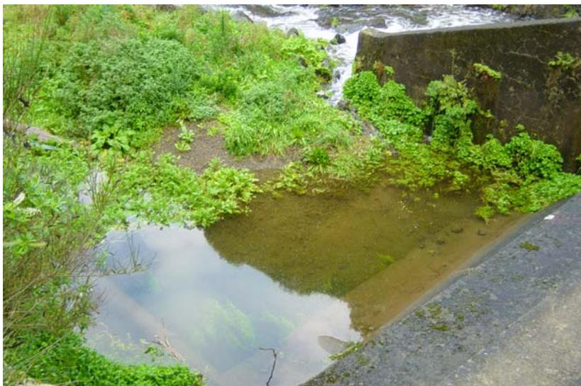
**Fig. B-29:** Right abutment – dam cast against rock.
