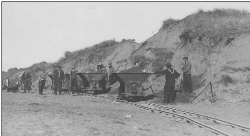
*Figure 4a and 4b: Large volumes of sand are being removed directly from Lyall Bay fore-dunes during the 1930s using tramways. Note the dense cover of sand-binding grasses on the dunes that are highly likely to be a mixture of spinifex and pingao (WCC archive photographs).*
