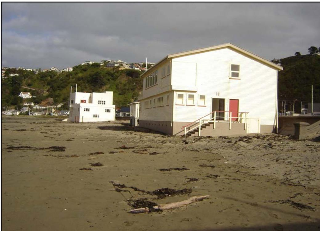
*Figure 13: AREA 5 showing buildings located seaward of the seawall that are clearly within the active foredune zone. The relatively flat beach is highly vulnerable to storm waves reaching the buildings and seawall.*
