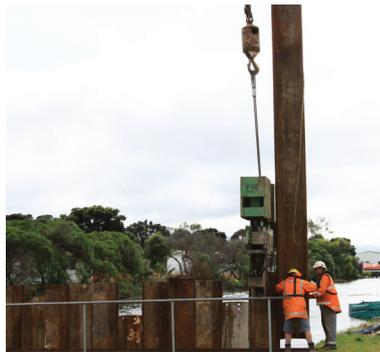
Collecting a sediment sample from the lower reaches of the Waiwhetu Stream for laboratory testing (left) and a pile rig at work installing the first sheet piles near the Bell Road Bridge (right).
