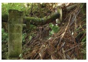
We replaced a vulnerable section of the water main to Karori, across the Kaiwharawhara Stream (pictured), with a new section of pipe buried beneath the streambed
