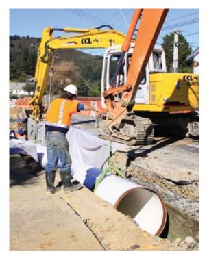
Diggers lift a new section of the Wainuiomata water main into place
