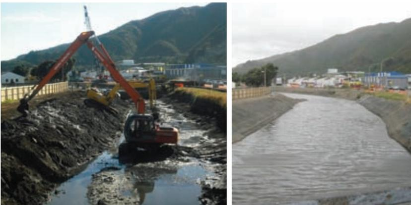
Diggers removing contaminated sediment from a section of the Waiwhetu Stream upstream of the Hutt Park bridge (left) and the same section of stream flowing naturally again and ready to be planted with native vegetation (right).
