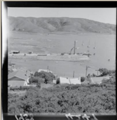
**Land reclamation at Paremata for railway (Main Trunk Line) including machinery, workmen, and boats on Porirua Harbour, Wellington Region.**
