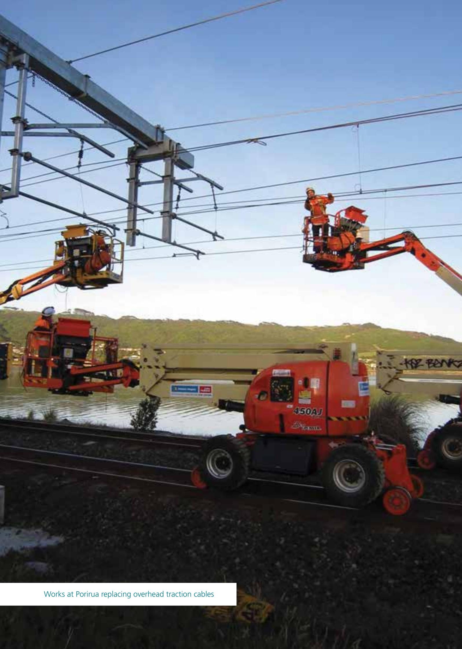
Works at Porirua replacing overhead traction cables
