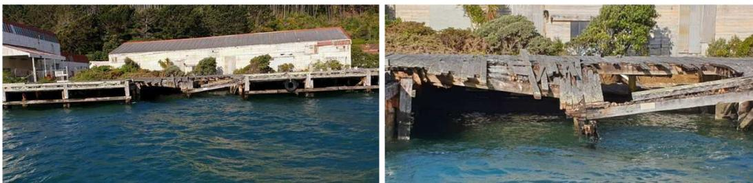
*Photograph One and Two: Pictures of collapsed Shelly Bay wharves.*
