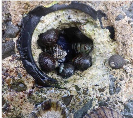
A weep hole in the surface of the existing new curved seawall at York Bay provides additional refuge areas for taxa when the tide is out.
