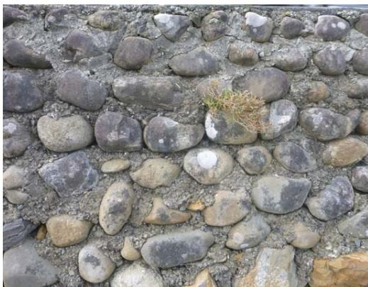
Concrete–aggregate wall with large cobbles set in place with concrete at Sorrento Bay
