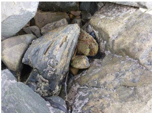
Revetment features cracks, gaps and a large surface.
