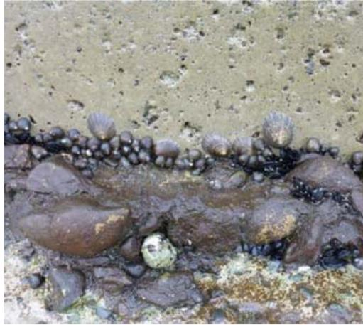
Larger substrate embedded in the toe of the existing new wall at York Bay provides additional habitat for biota.
