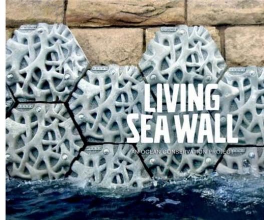
A 3D printed seawall texture that is being trialled in the Sydney Harbour as a living seawall.
