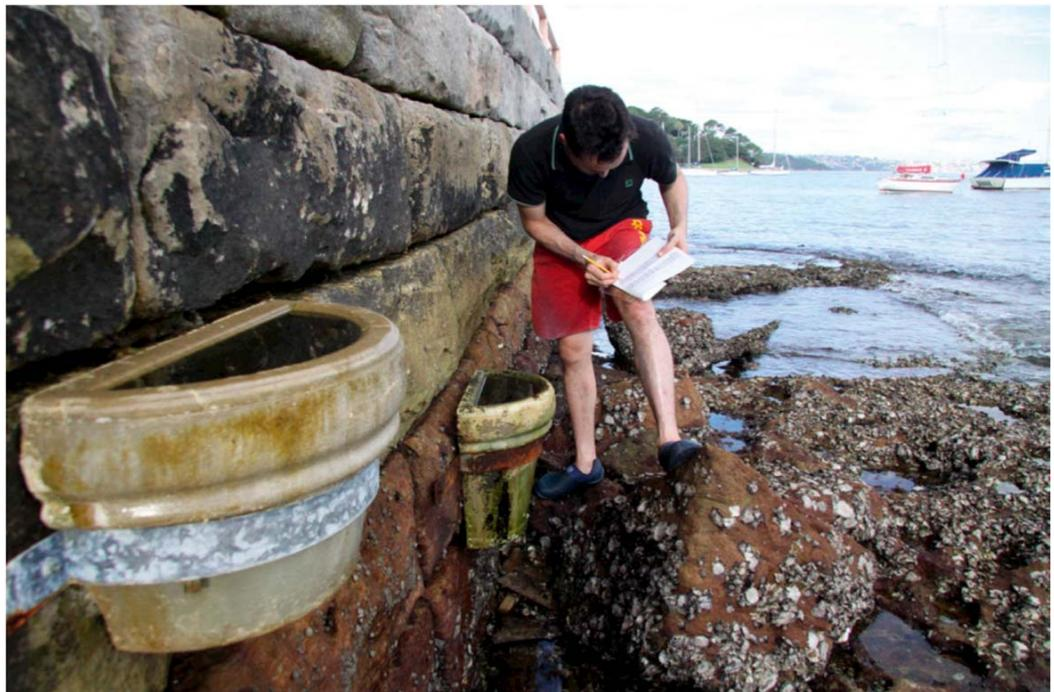
Figure 40 Example of a 'window box' rock pool on a flat vertical face from Chapman & Browne (2014).
