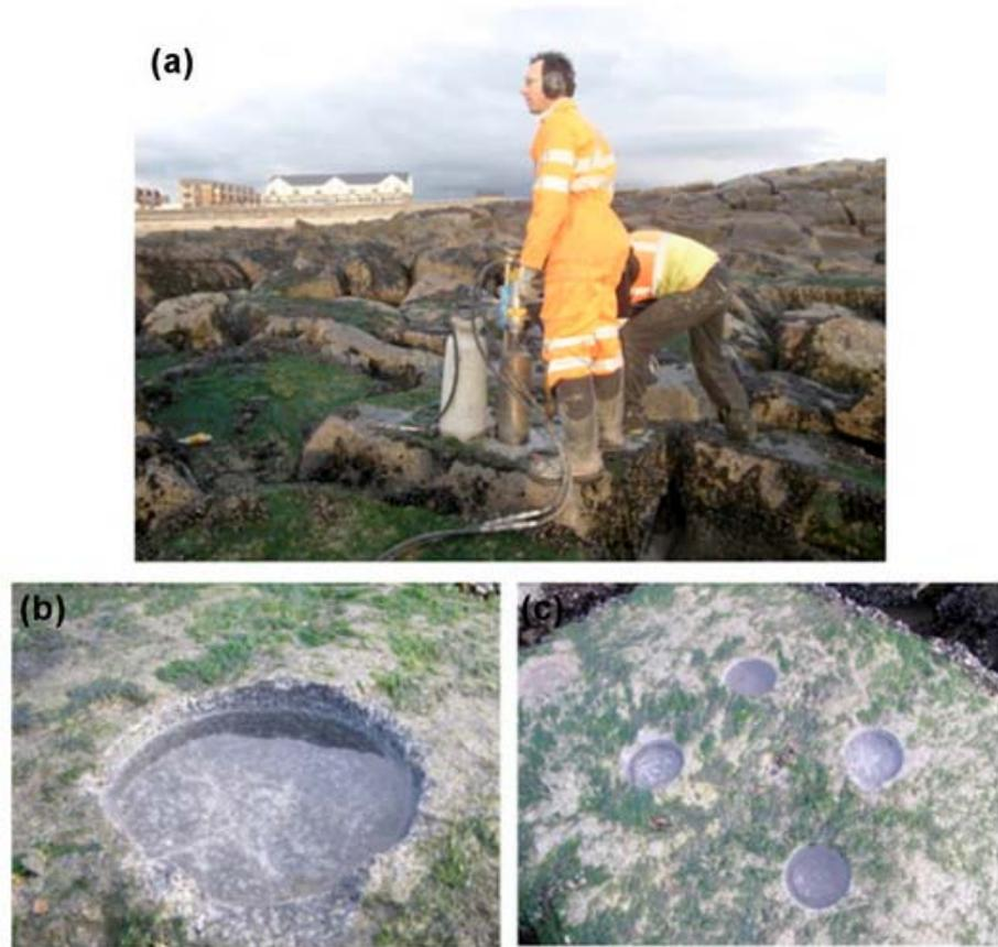
**Figure 4.11** Drill-cored rock pools at Tywyn, Wales. (a) Contractors drilling the pools in November 2011. (b) Shallow (5 cm deep) pool. (c) Four pools on the surface of a boulder. All photographs by L. Firth.
