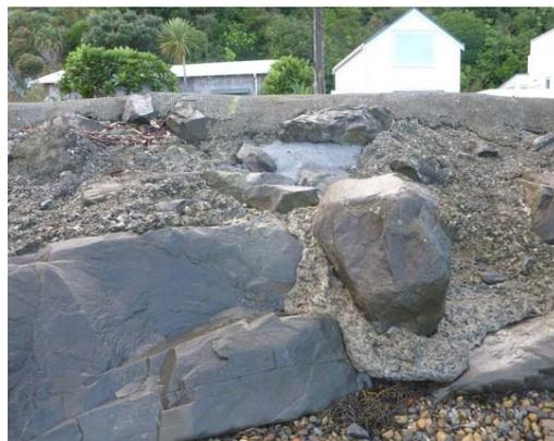
Concrete–aggregate seawall at Mahina Bay where concrete has been poured around boulders
