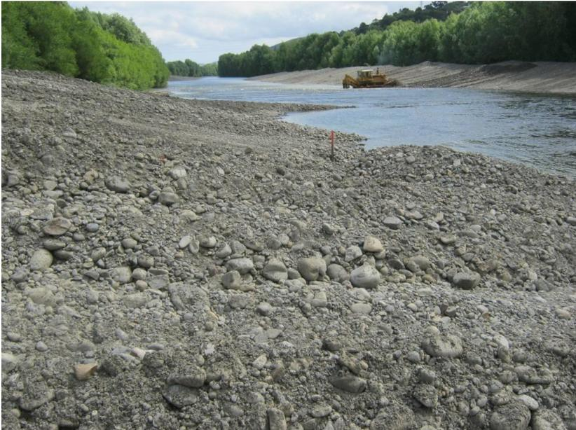
Figure 10: 'Wet' gravel extraction: bulldozer forming low flow channel
