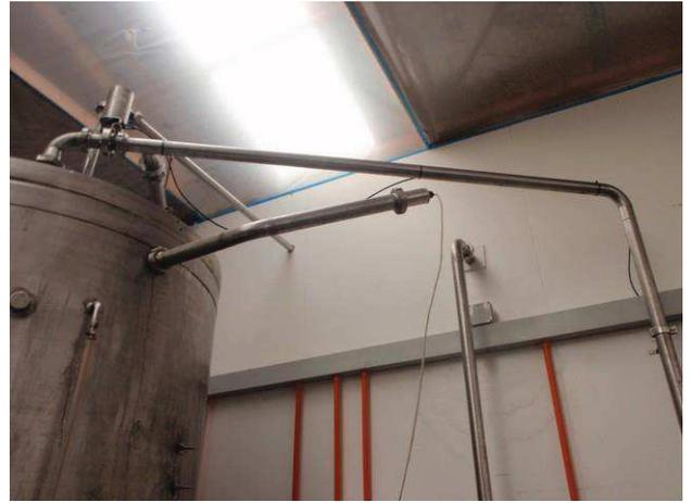
**Figure 6 & 7:** Pipes transferring water past the meter to the storage tank.
