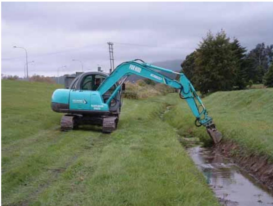
**Figure 5-8:** Stormwater drain clearing in the Hutt catchment
