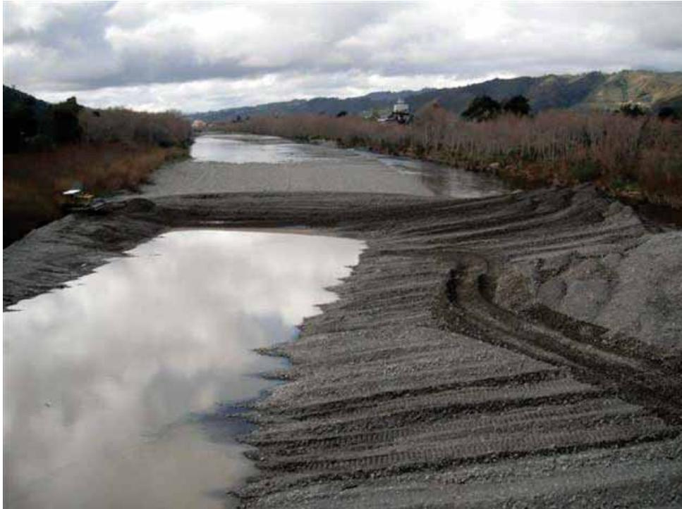
**Figure 5-10:** Gravel extraction; shaping of a new low flow channel with meander pattern
