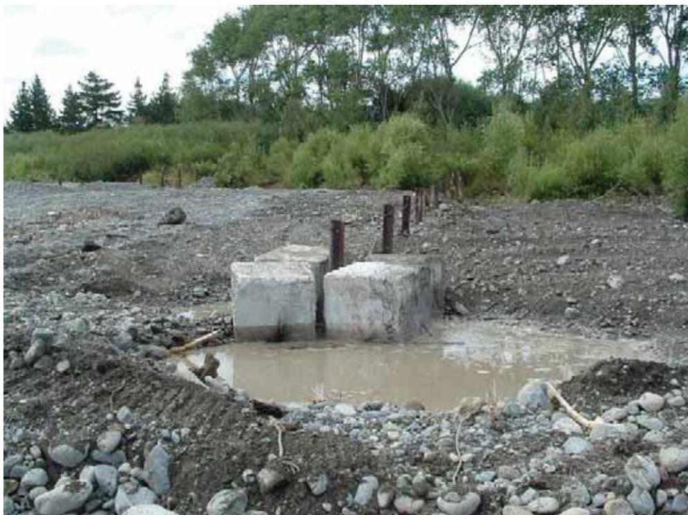
**Figure 5-6: Completed debris fence (Otaki River)**
