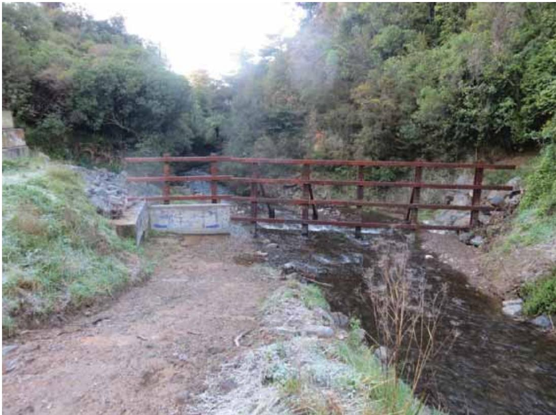
Figure 3-12: View of the debris arrester on Speedy's Stream
