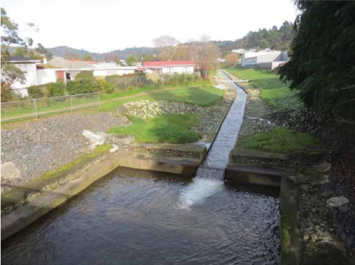
**Figure 3-5:** View of concrete lined channel and stilling basin at Stokes Valley Road, within the application area
