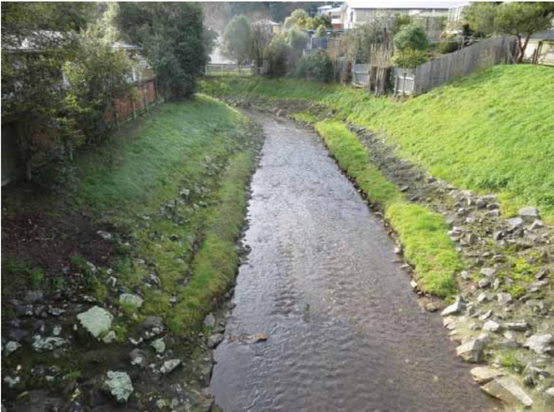
**Figure 3-6:** View of modified straightened stream channel downstream of Stokes Valley Road, within the application area
