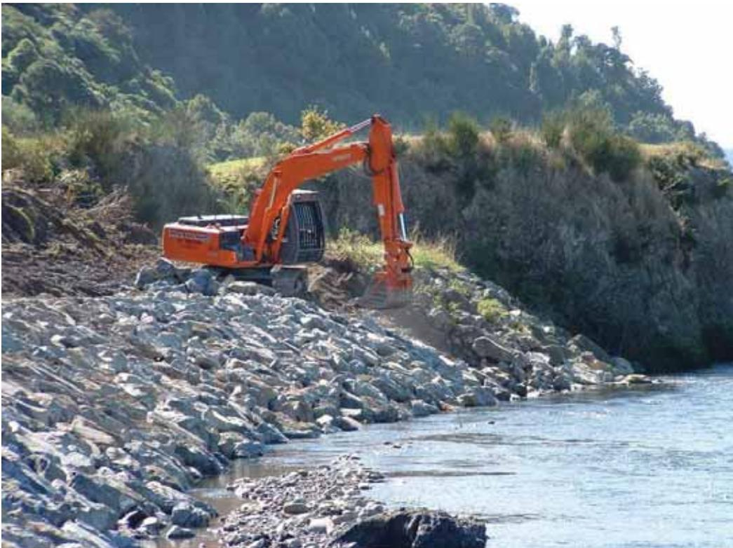
**Figure 5-5: Construction of rock rip-rap lining on the Hutt River**
