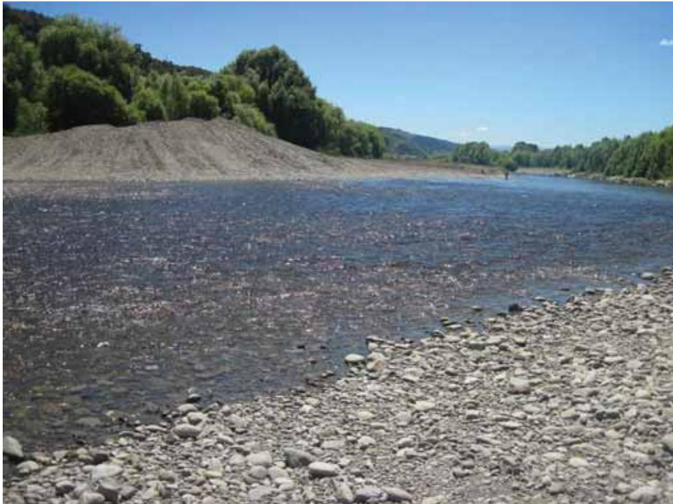
**Figure 5-11:** Riffle on 20<sup>th</sup> December 2012 near Kennedy Good Bridge, one day after completion of gravel extraction and channel shaping works, showing simplified channel structure and reduced substrate particle size (compared with pre-works)
