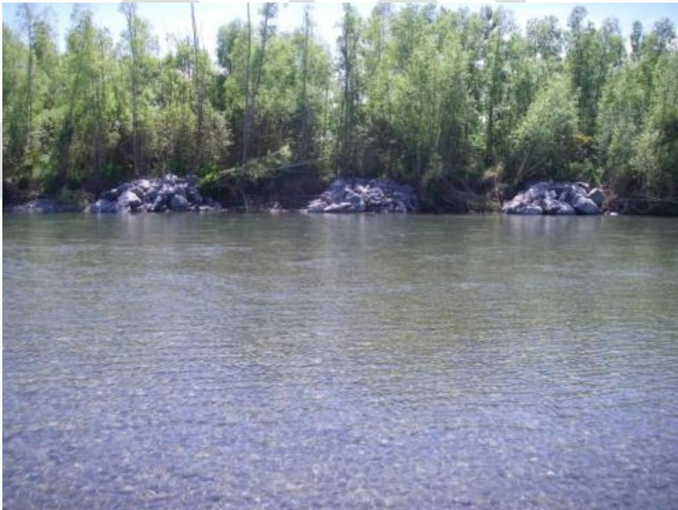
**Plate 12:** Waiohine River at river works area with rock groynes in place.
