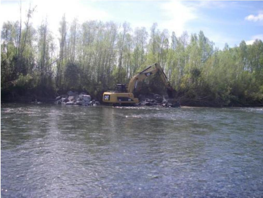
**Plate 7:** Rock groynes being placed in a stretch of the Waiohine River in 2012.
