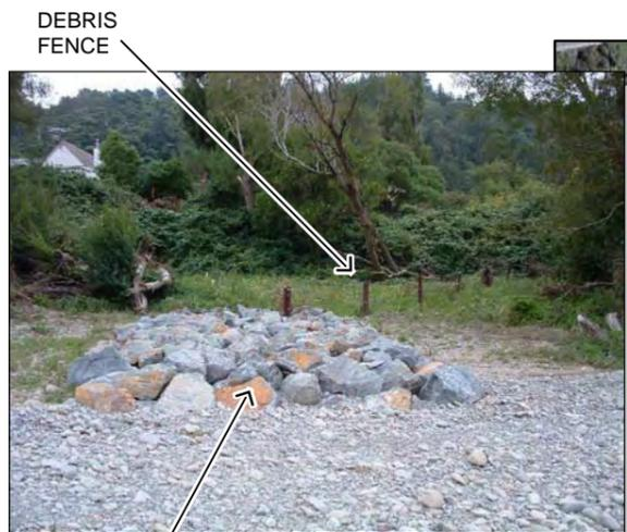
PHOTO OF DEBRIS FENCE WITH ROCK HEAD
