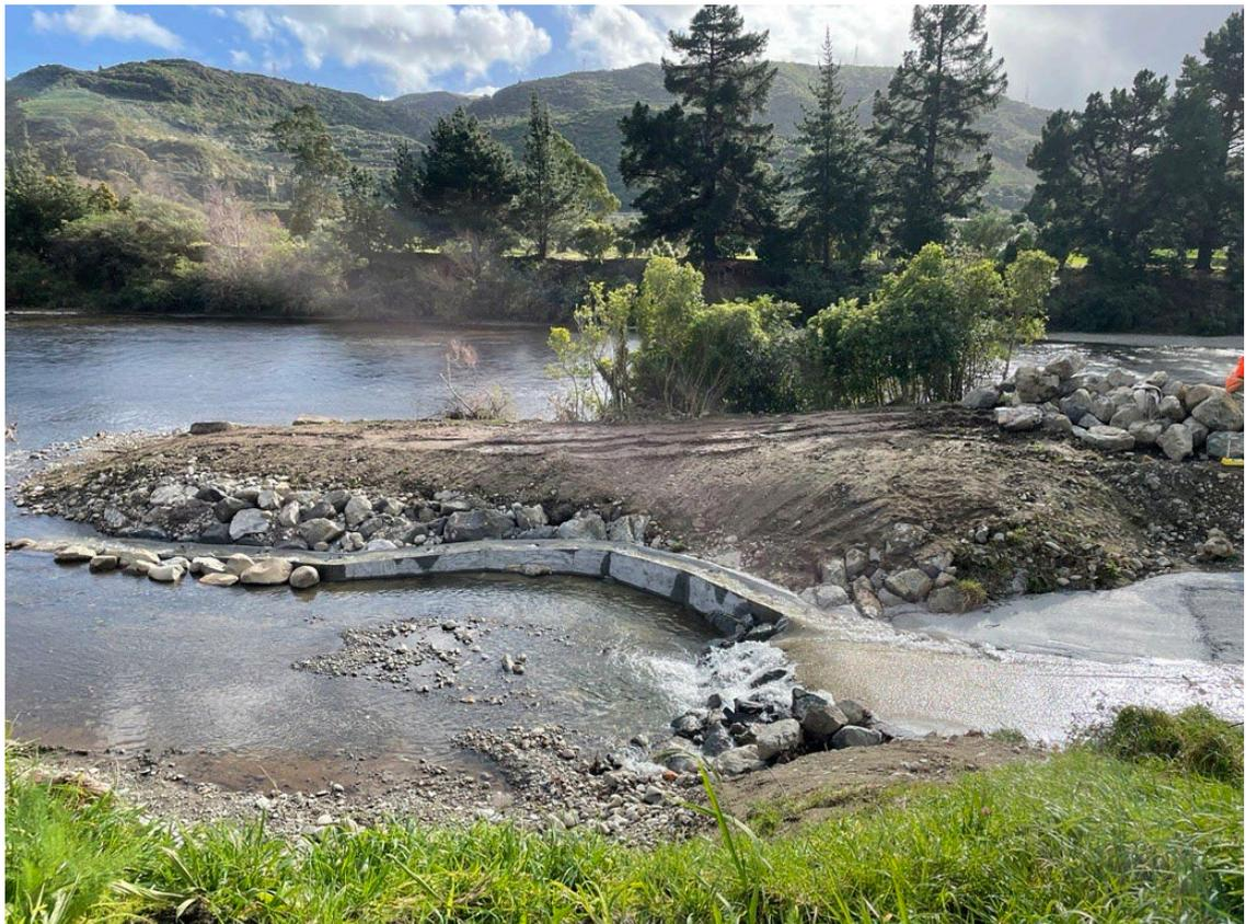
*Figure 5: Site 1 - Stokes Valley Stream fish passage and repaired weir*
