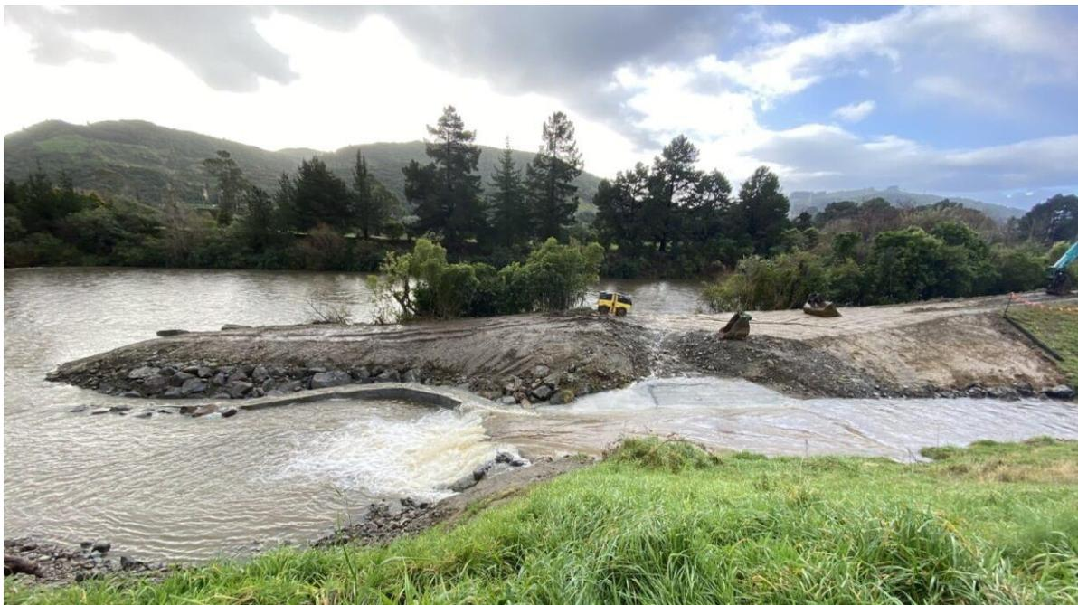
*Figure 1: Stokes Valley Stream mouth showing the stream diversion and reinstated training bank*
