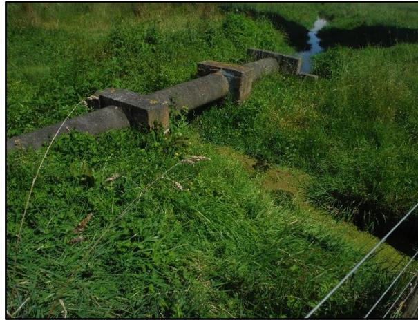
**Figure 12: Site 18 Piped water race section crossing over a natural stream, March 2023.**
