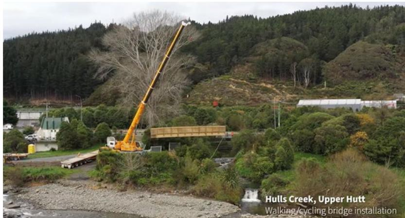
**Figure 4: Hulls Creek Bridge installation**
