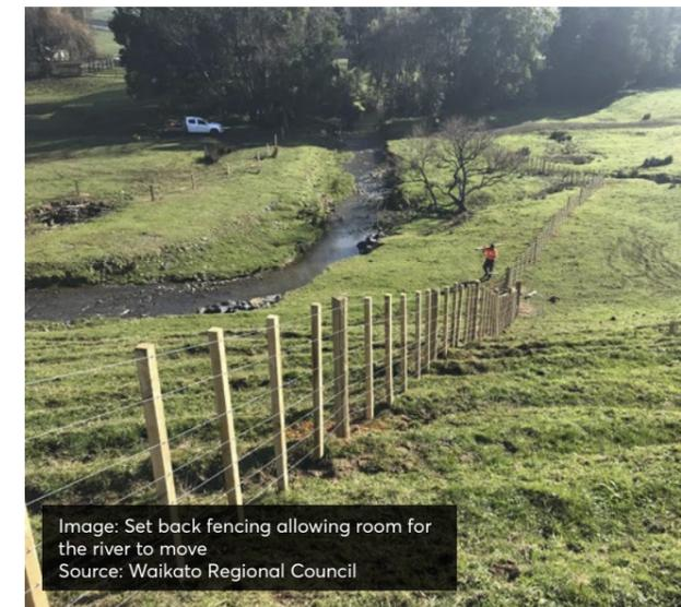
Image: Set back fencing allowing room for the river to move
