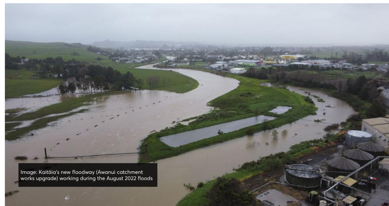
Image: Kaitāia's new floodway (Awanui catchment works upgrade) working during the August 2022 floods
