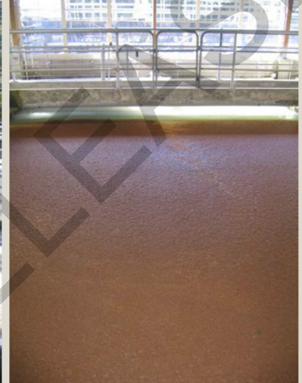
Float layer over filter
