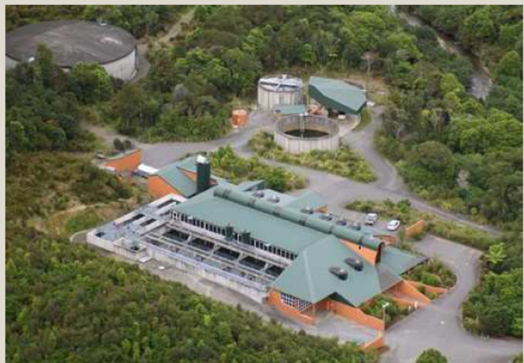
Wainuiomata Water Treatment Plant
