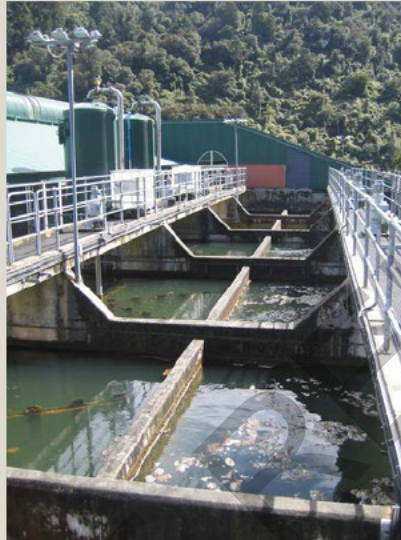
Flocculation tanks
