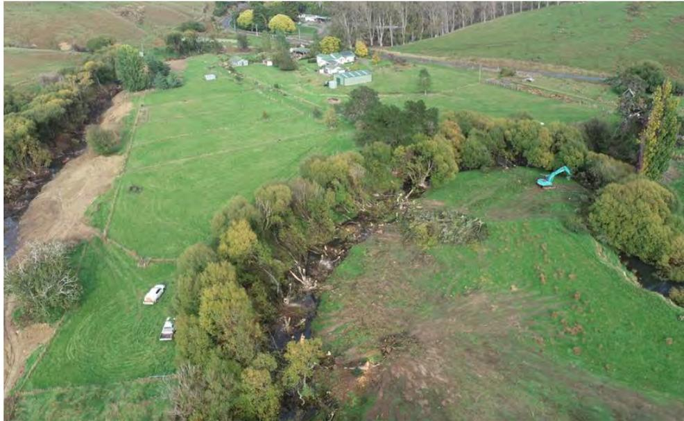
*Figure 2: Whangaehu River – Large blockage area within the upper reach (during blockage removals)*
